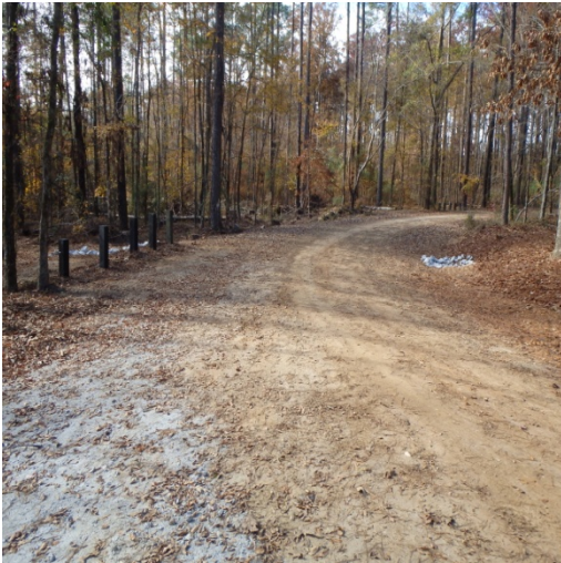
Main road needs culvert or low water crossing
